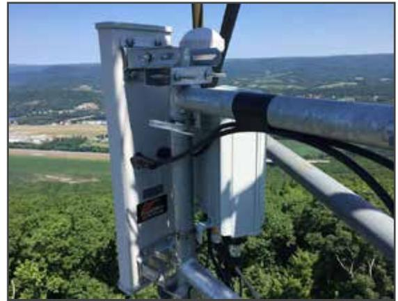
*Figure 6: Baicells Nova R9 1 Watt Base Station with Antenna*
